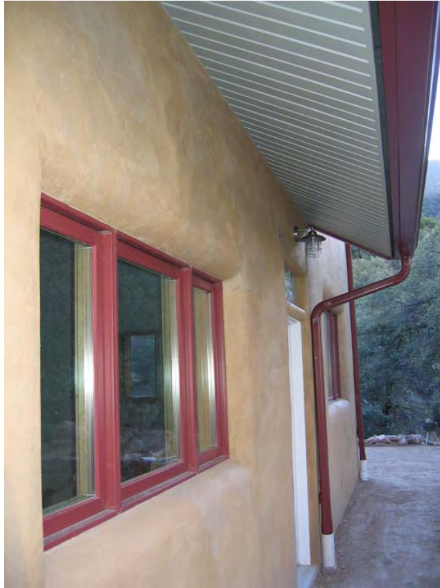
Photo E.4. Firewise windows, door, and soffits
