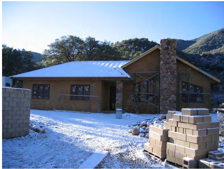
Photo E.2. Firewise home construction
